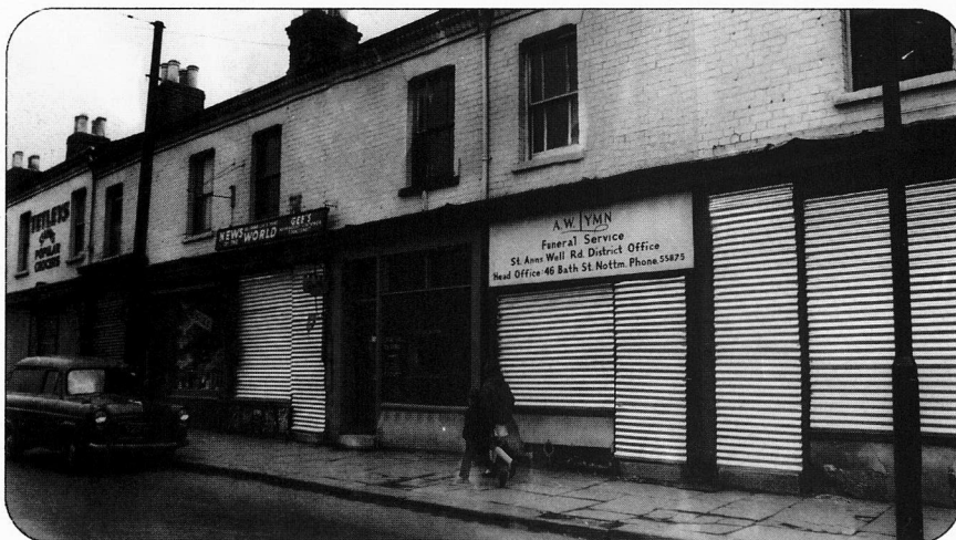
Some of the "tinned up" shops on St Anns Well Road (near Robin Hood Chase) await demolition
