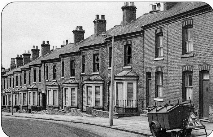
Doomed houses in Hungerhill Road await demolition. In the foreground is a handcart belonging to one of the gangs travelling around the area turning off power supplies
