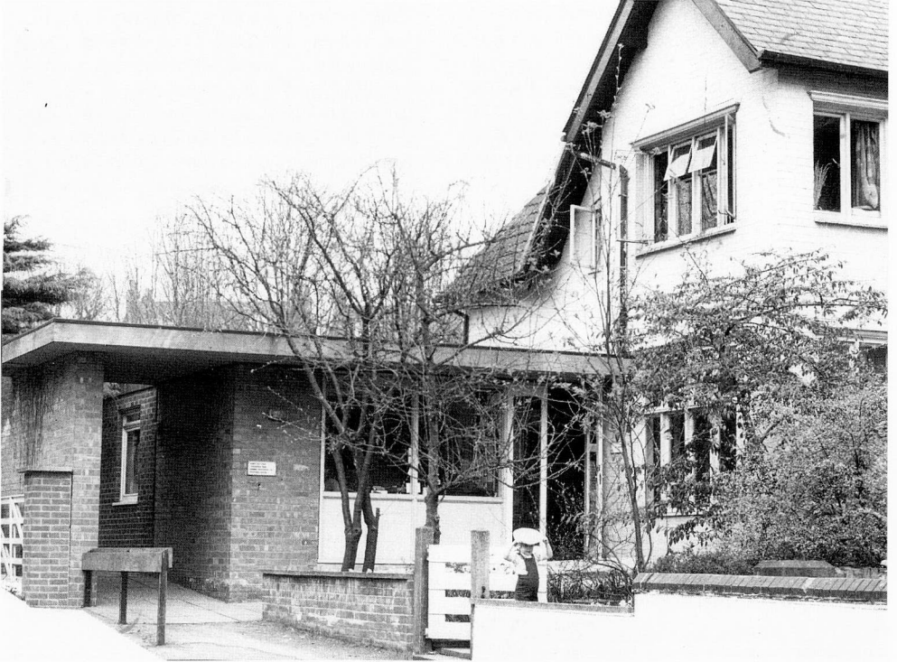
Soon after The Croft opened, this small office extension was built to cope with the large demand for Family First's help. The Croft remained Family First's administrative base for more than three decades. The open front door led to the Reception office on the left and the large Community Room on the right. A coin telephone in the lobby was used by neighbours and tenants. See chapter on Neighbourhood Centres
