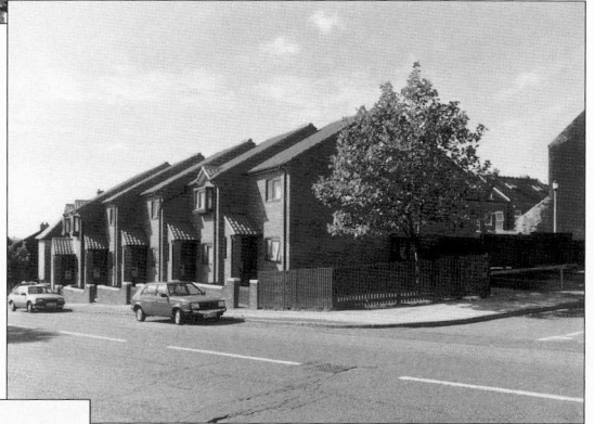
Houses completed in 1990 by Family First in St Ann's, Nottingham
